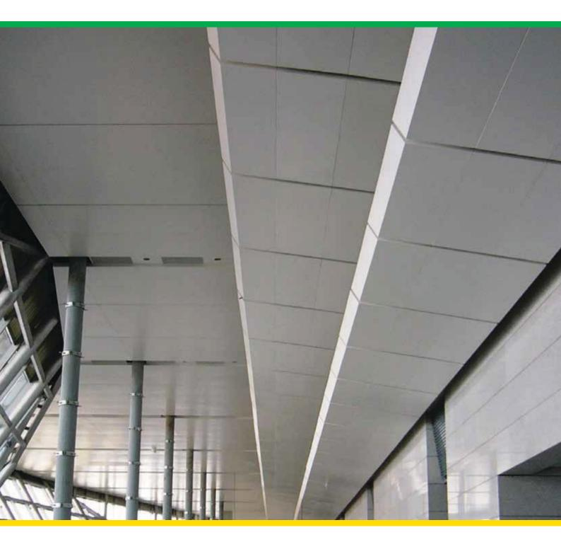
The USG Boral Honeycomb Ceiling System is lightweight and easy to install and demount. The system has an aluminium core with either a powder coated or PVF2 treated aluminium face panel which is adhered to the back aluminium layer. The USG Boral Honeycomb Ceiling System is available in different color, height and edge options to meet customized needs.
